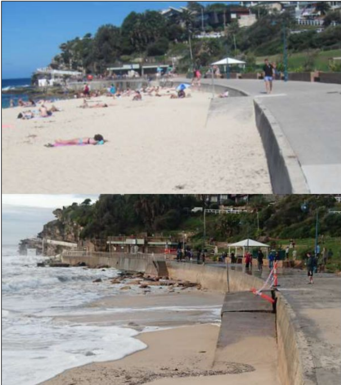
Figure 5-10 View of southern length of Bronte Beach and seawall showing differences in beach profile before (top image, 1 April 2016) and immediately after (bottom image, 6 June 2016) the East Coast Low storm event (source: (ARUP, 2016) (top), (Baird, 2016) (bottom)).
